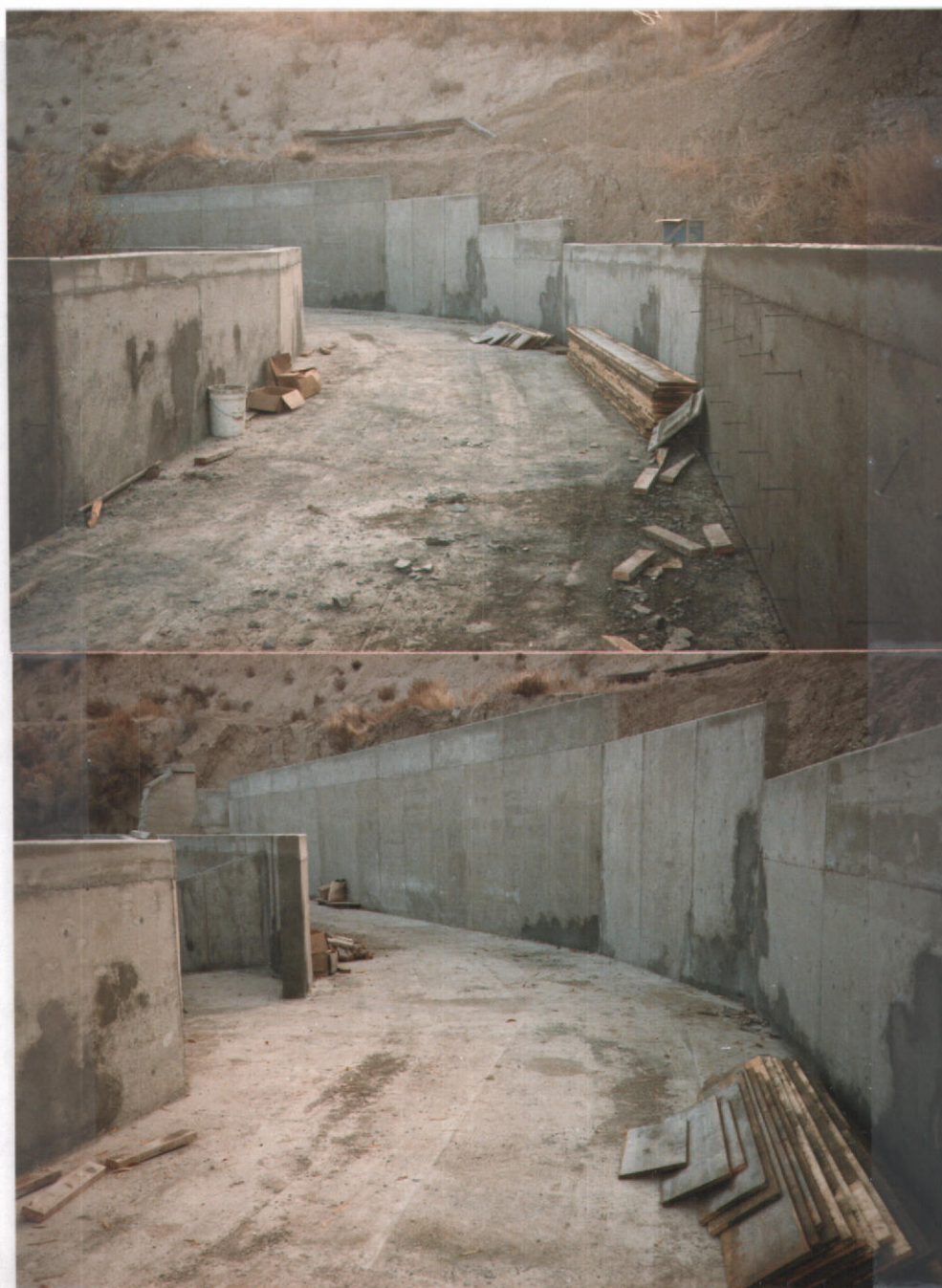
Diversion Canal Under Construction
