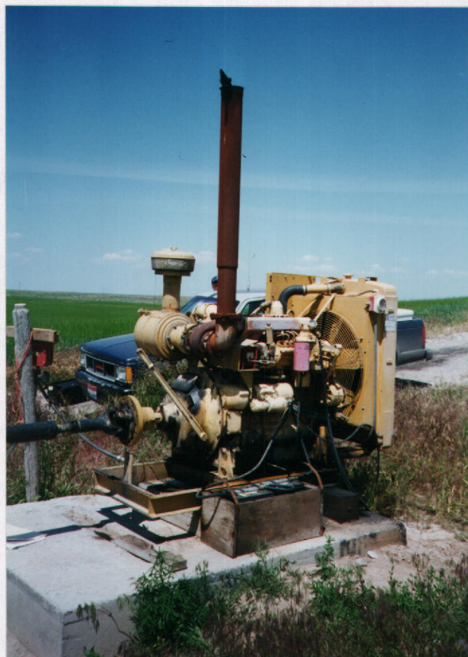
Plate 2 - Closeup of Cat 3304T at point of diversion.
