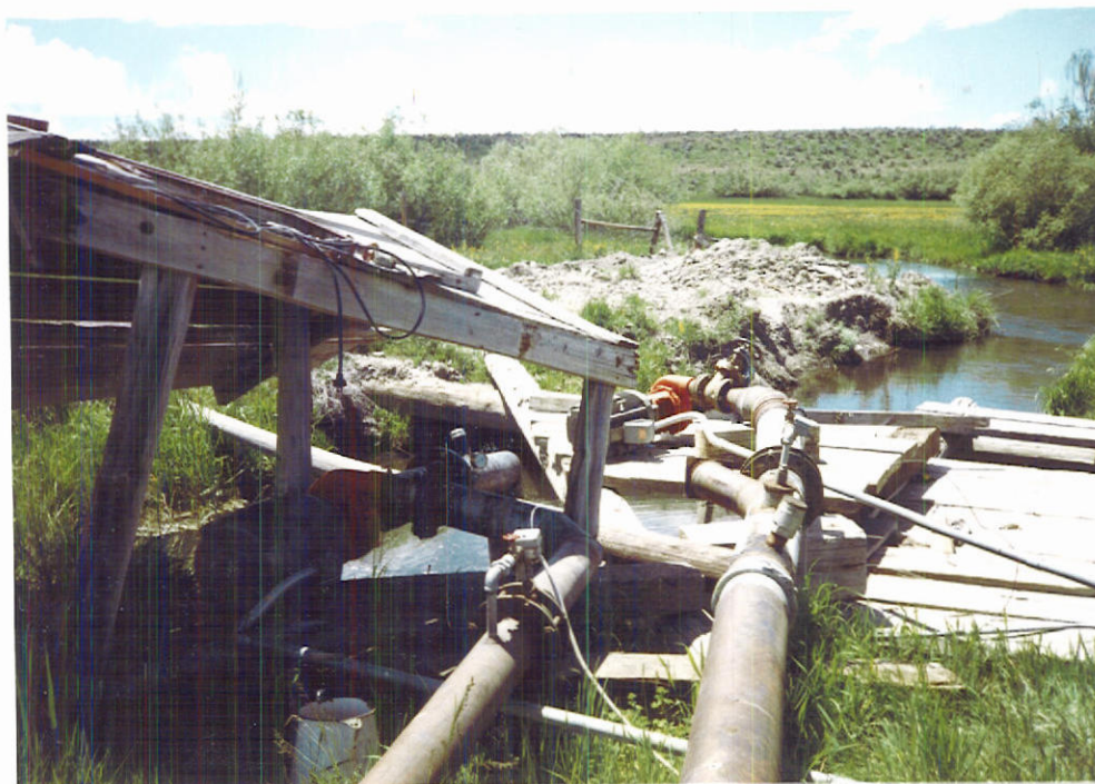
Close Up of Pumps, 8" Piping and Valves
