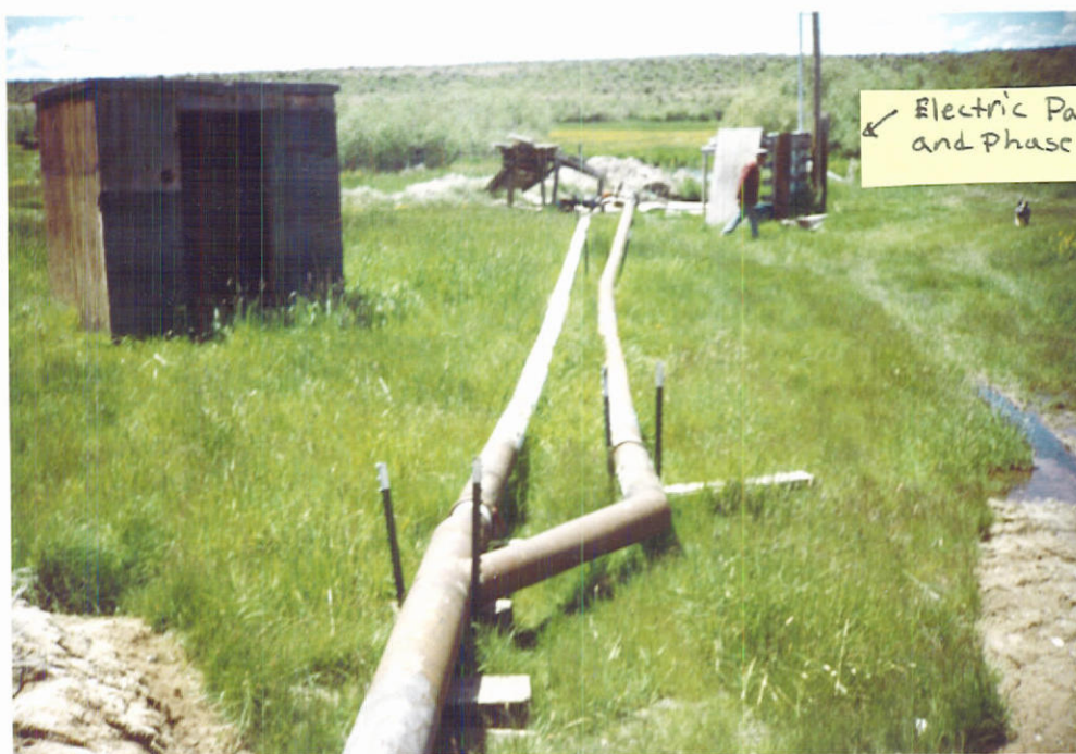
2 - 8" Lines from pumps Join Into 10" Main Line Distance from pump to joint - 45 ft.
