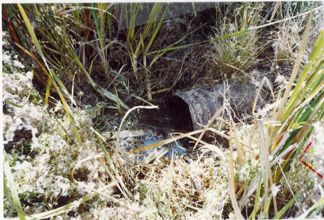
North of Highway 78 Looking South- east at North end of the culvert that runs under the highway
