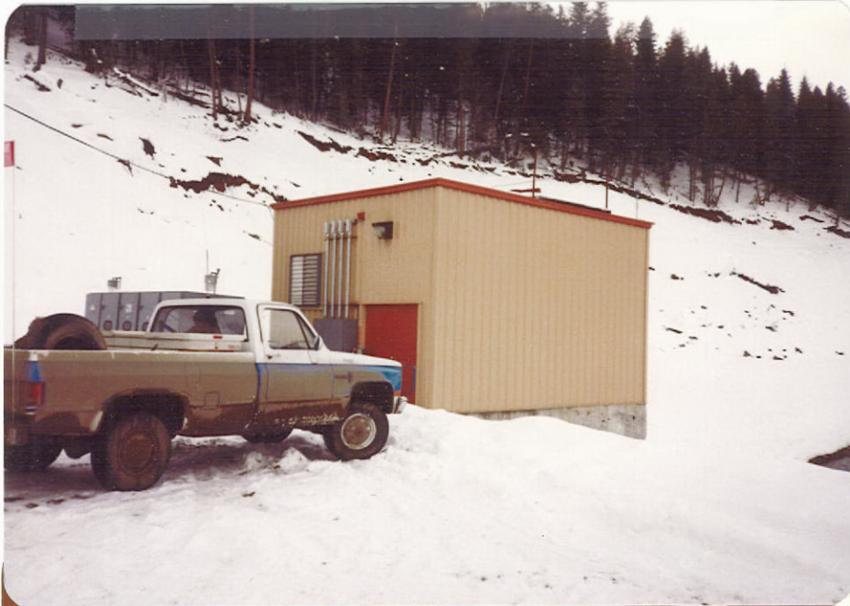
Seepage return Pumphouse
