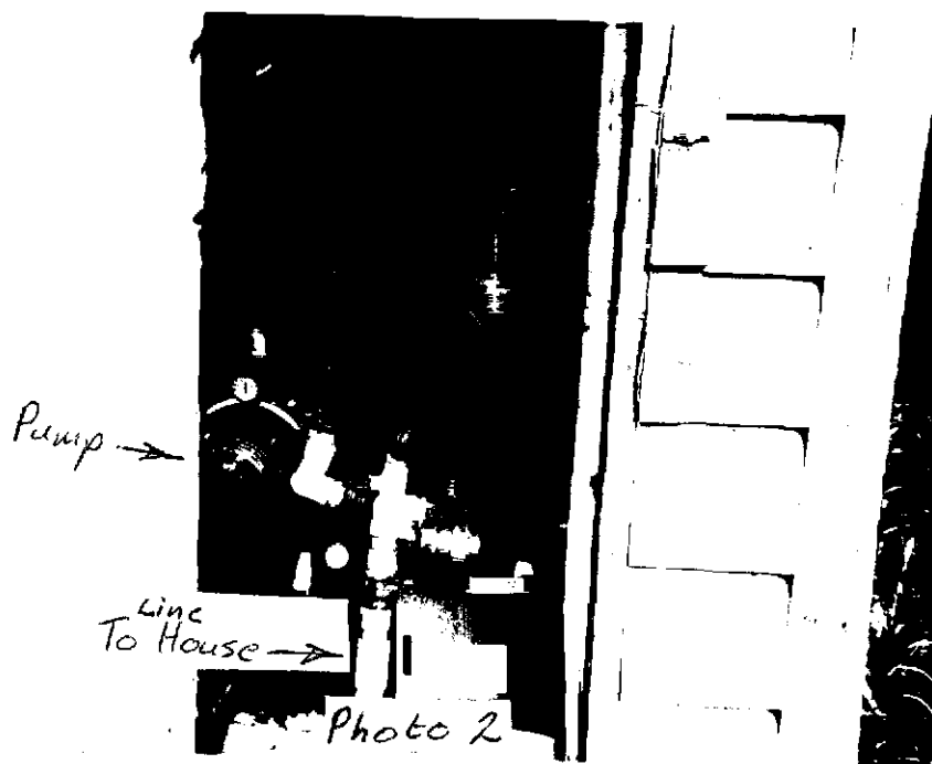
Photo 2. Showing Inside Pump House.
