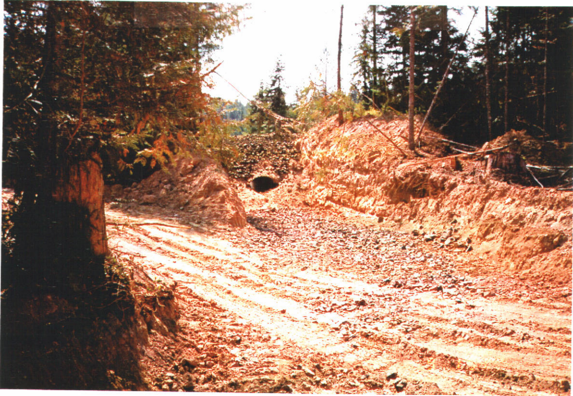
Looking down the spillway channel toward the culvert under the access road to Needhams house.
