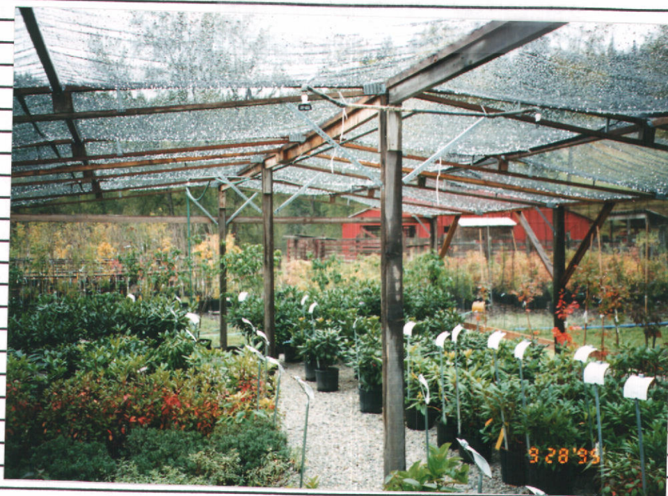
* SHADE HOUSE WITH OVERHEAD "MIST TYPE" SPRINKLERS.
