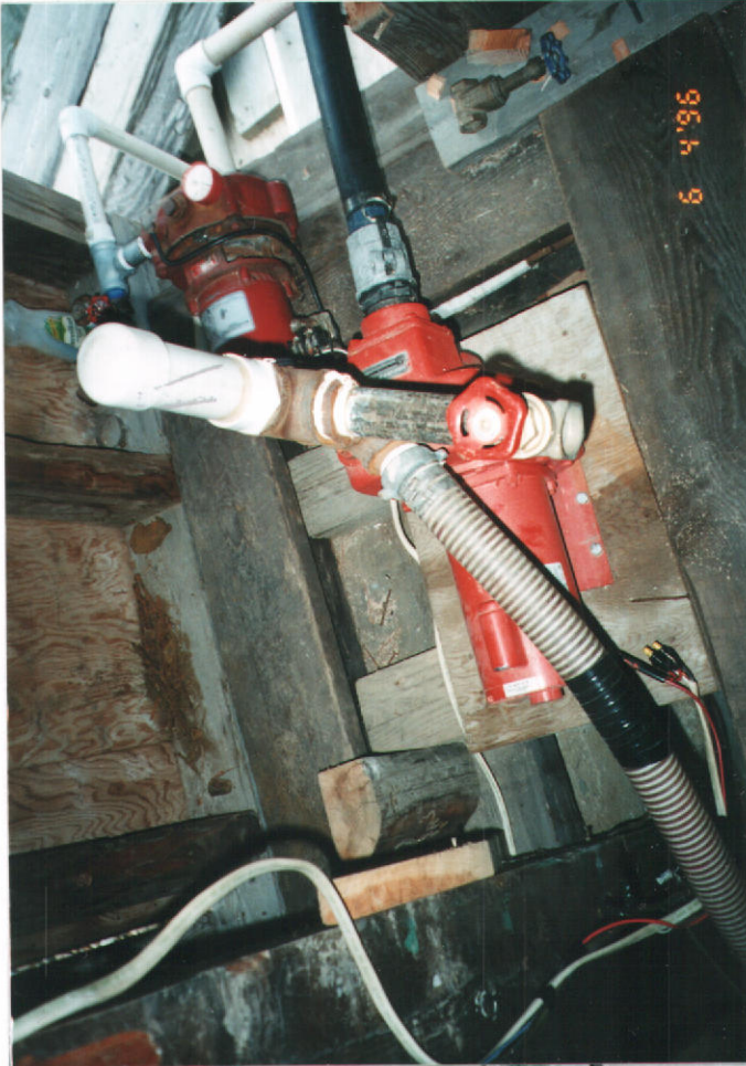
FRANKLIN 2 HP PUMP PUMP SITE
