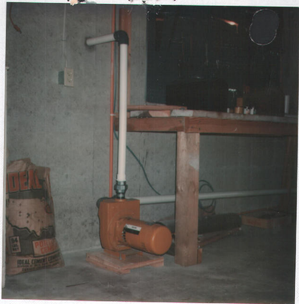
Pump installation for J. H. Gridley photo taken February 21, 1976
