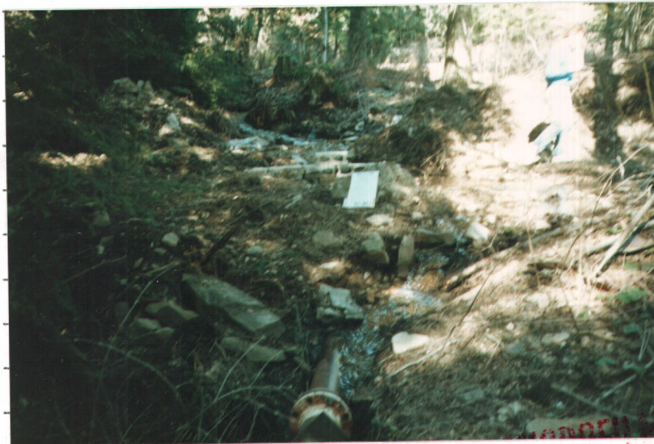
6" STEEL CASING TO 2" PIPE
