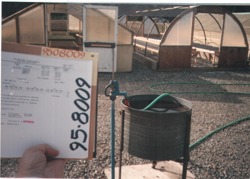
TYPICAL FROST FREE RISER
