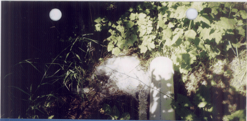
Discharge Top of Water Feature
