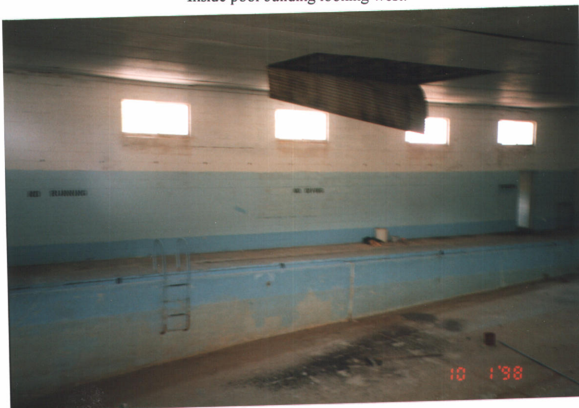
Plate 4 – Bear Lake Hot Springs. Inside pool building looking north west.
