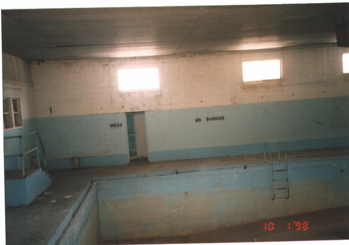
Plate 3 – Bear Lake Hot Springs. Inside pool building looking west.
