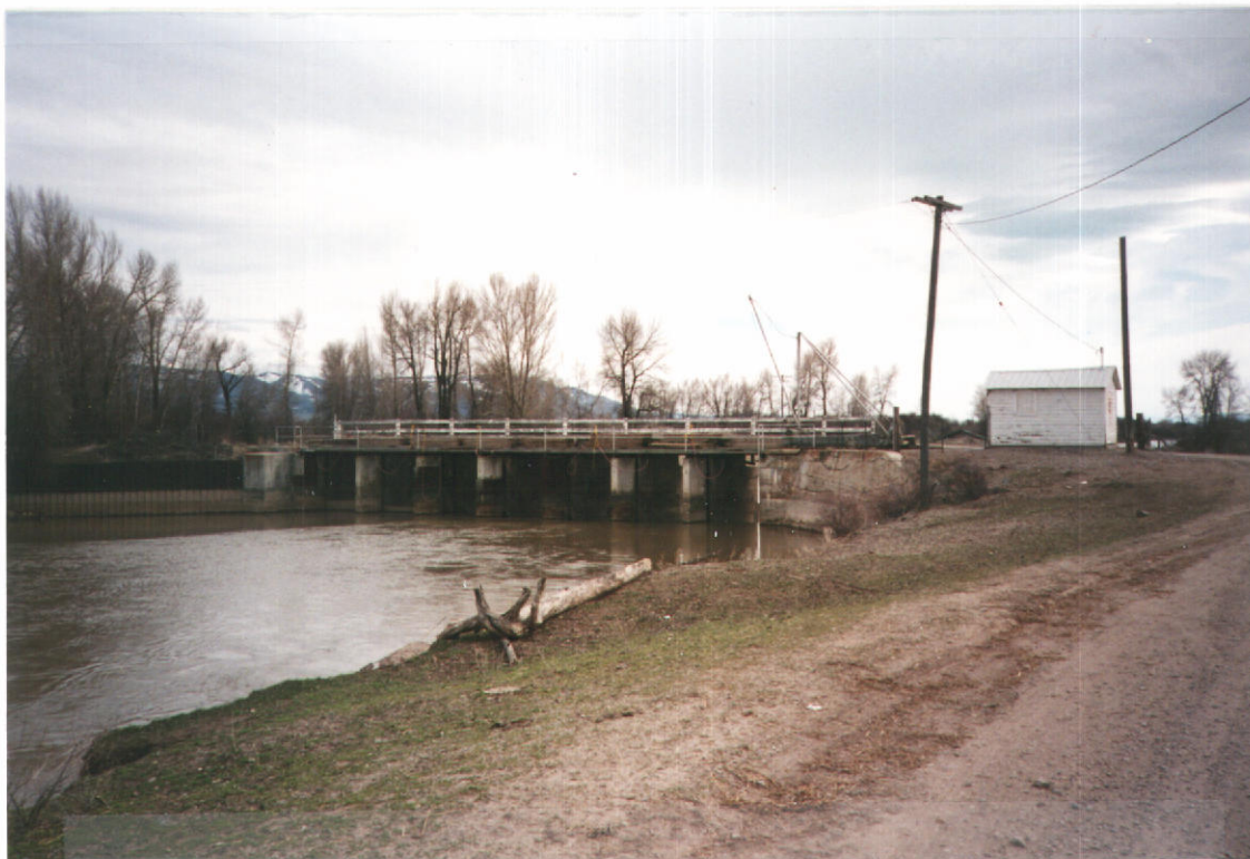
Fig. 2 - Controlling headworks of Rainbow Inlet Canal.
