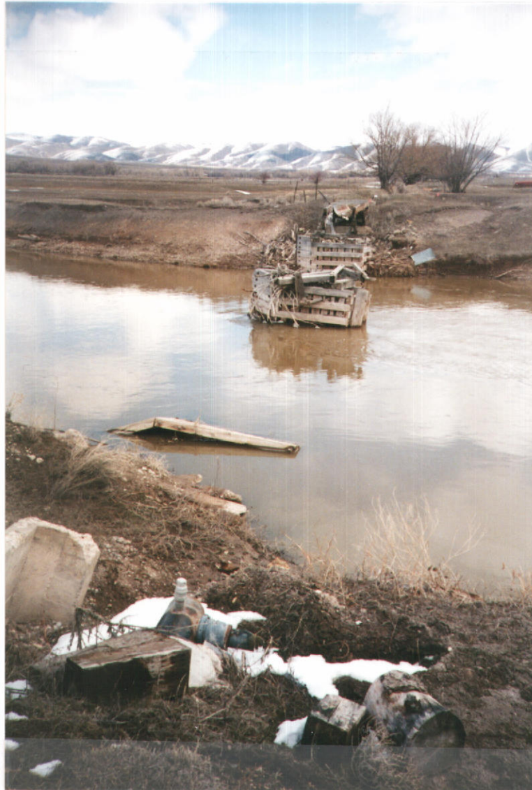
Fig. 3 - Site for pumping station in Rainbow Inlet Canal.
