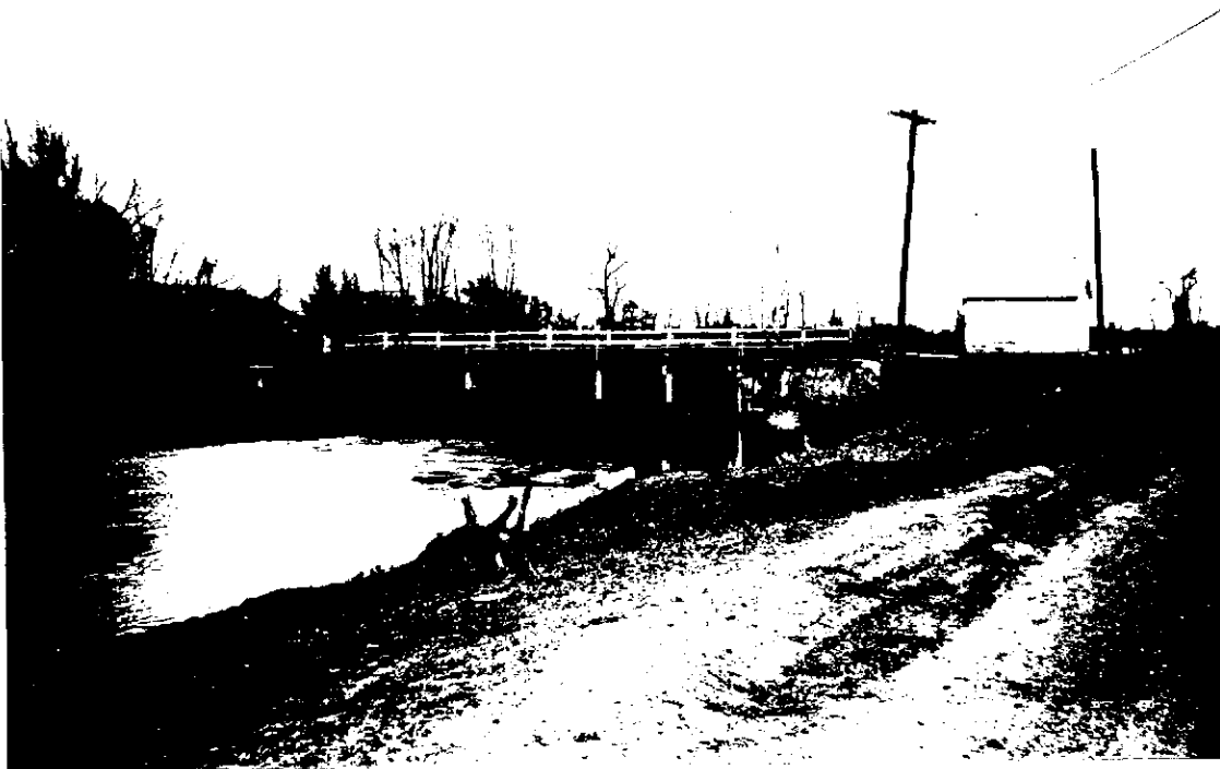
Fig. 2 - Controlling headworks of Rainbow Inlet Canal.
