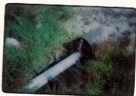
Culvert near highway
