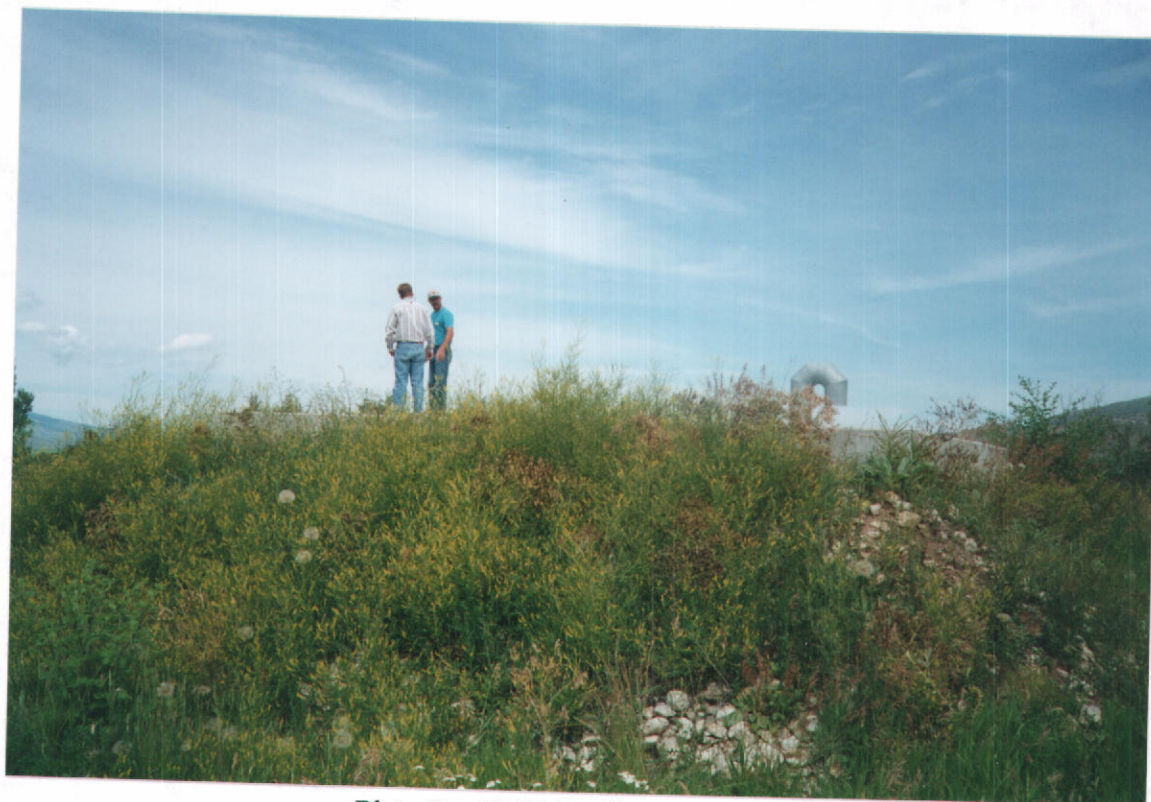
Plate 2. - 50,000 gallon storage tank for Townsite of Bennington. MICROFILMED
