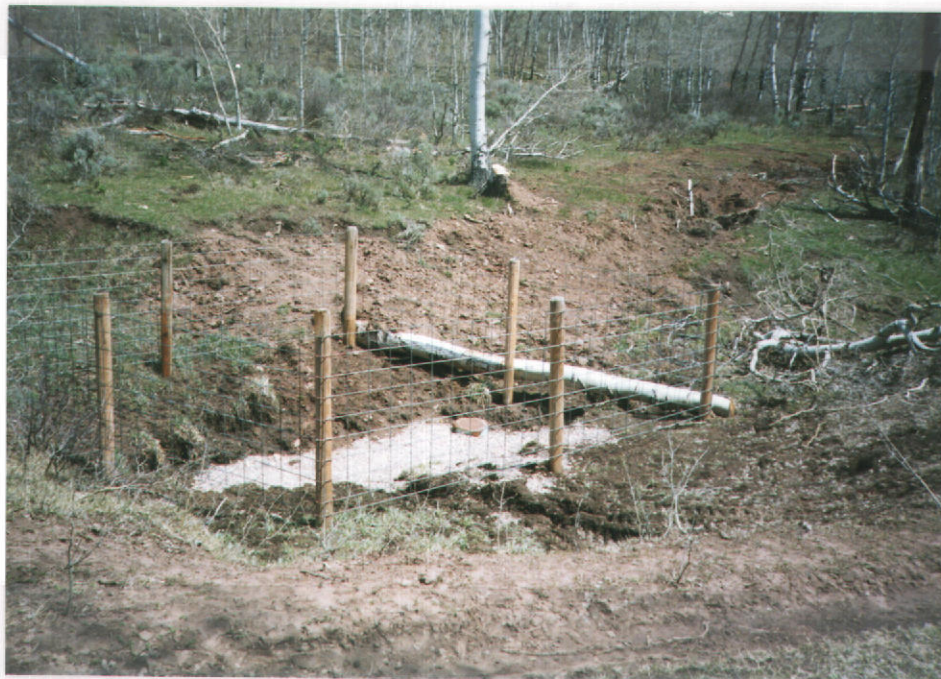
Fig. 1 - Point of diversion at spring showing enclosure.
