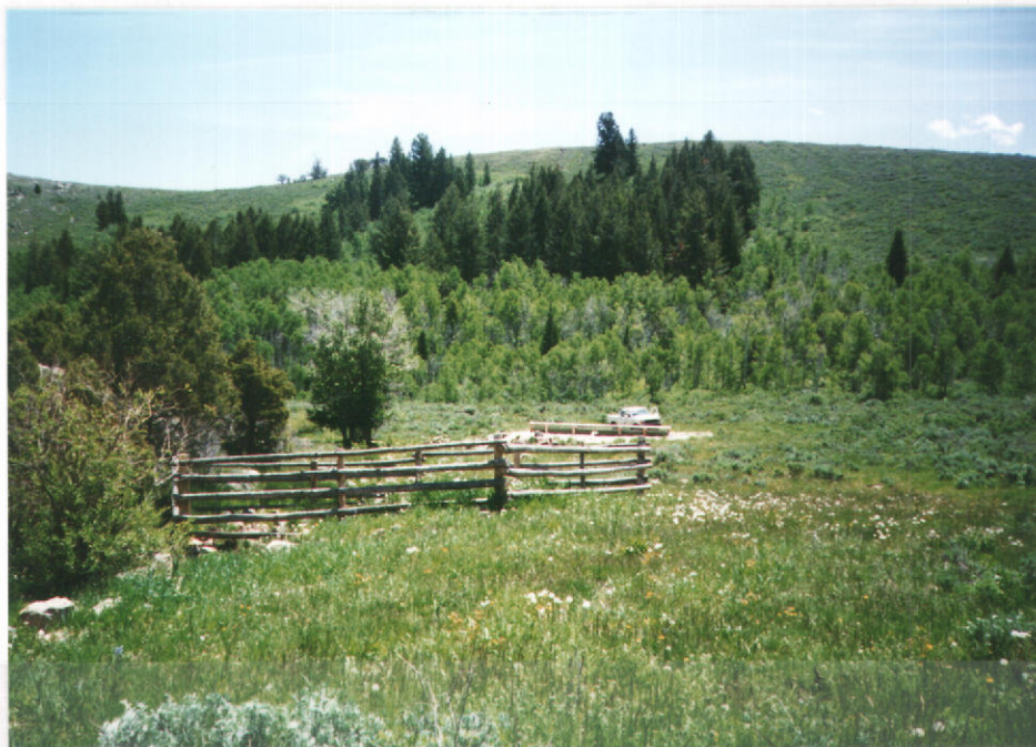
Fig. 2 - Complete system showing spring enclosure. and stockwater trough.
