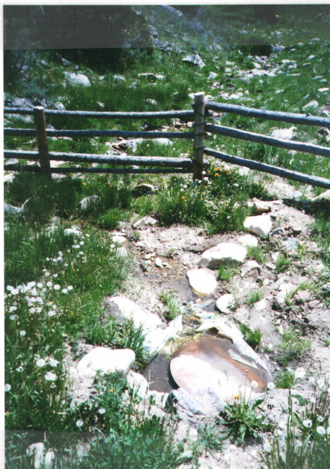
Fig. 1 - Point of diversion showing springbox.
