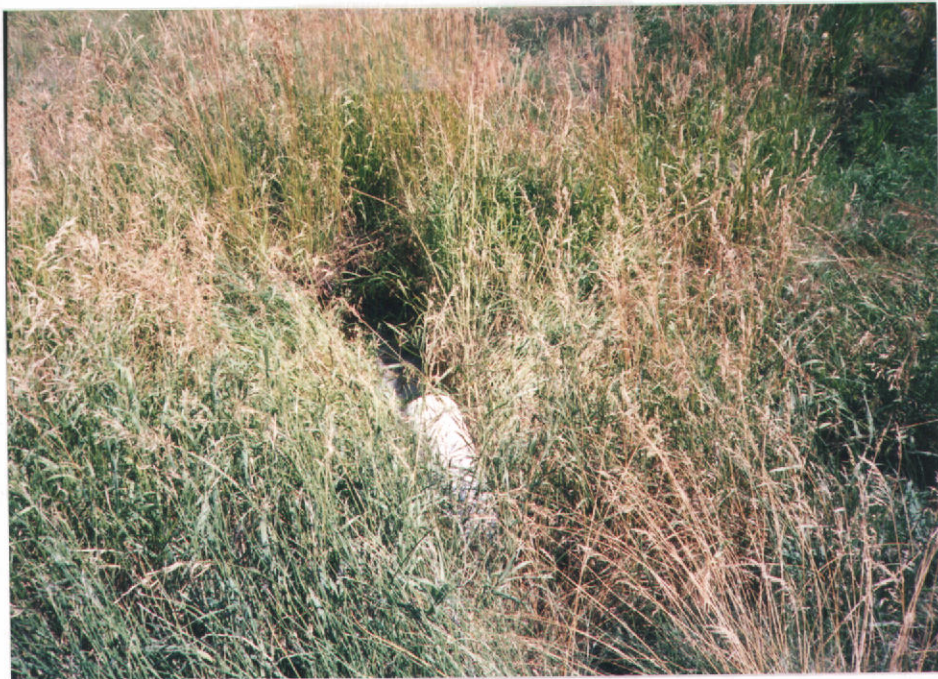
Looking North East a outlet pipe and open channel back Permit # 11-7431 to Bailey Creek
