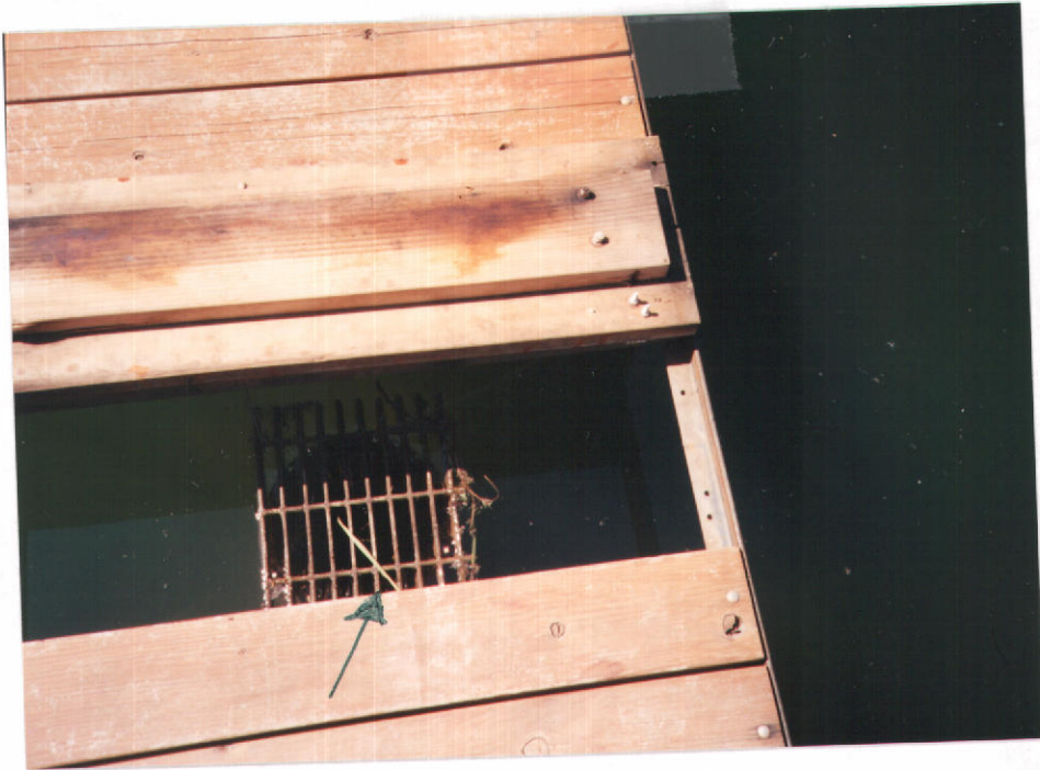
Looking down on outlet Screen
