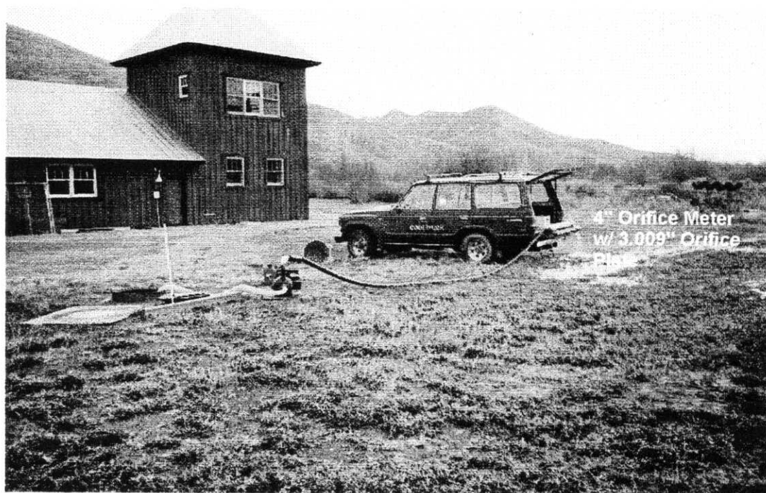
Pumping sump to determine system capacity.
