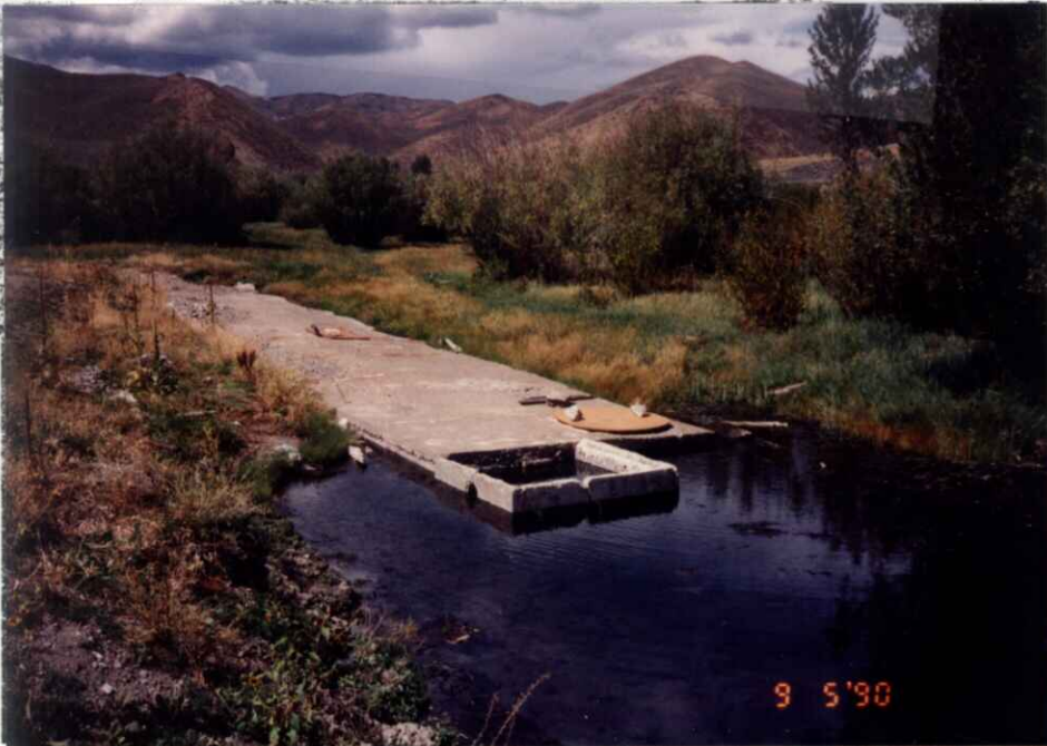
old cistern in hot water system
