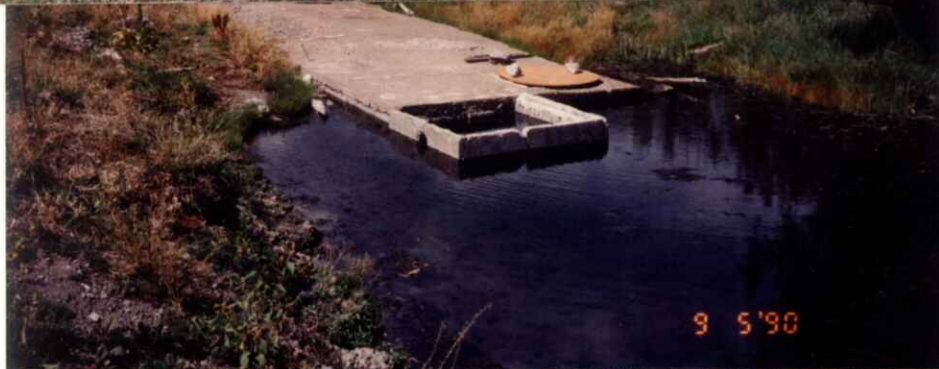
Developed spring box above concrete cistern
