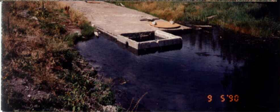
Developed spring box above concrete cistern
