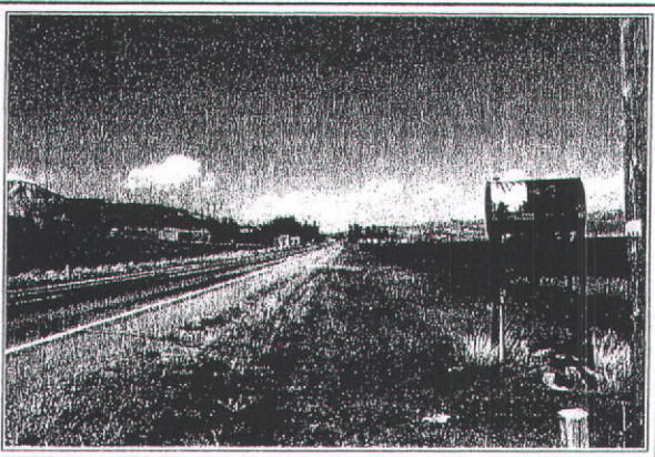
West Side Highway Along a Portion of the West Property Boundary
