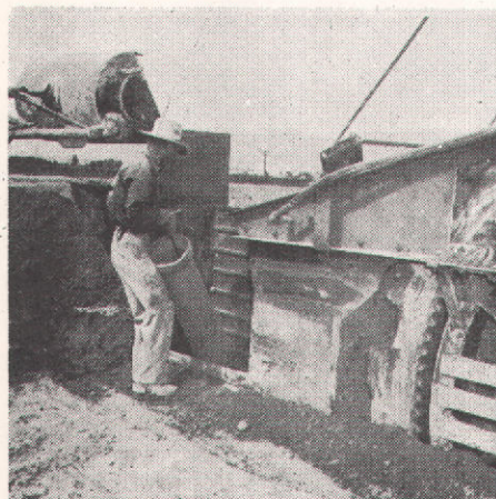
Top—Machine to dig trench, lay pipe and apply gravel filter in one operation is invention of the late Sumner G. Margetts. Device is manufactured at Layton shop.
