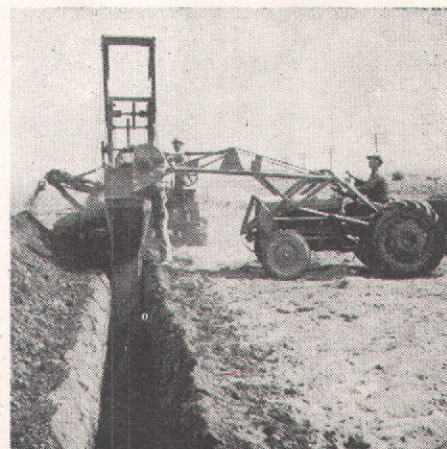
Top—Machine to dig trench, lay pipe and apply gravel filter in one operation is invention of the late Sumner G. Margetts. Device is manufactured at Layton shop.
