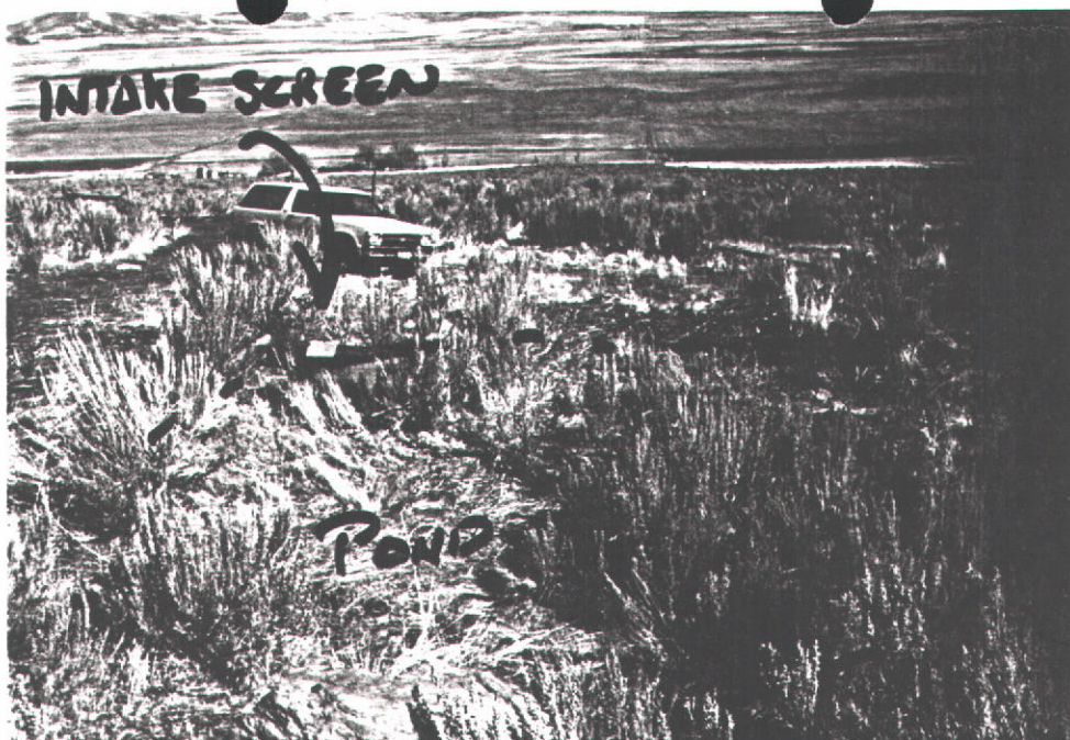
DOWNSTREAM VIEW OF DIVERSION IN UNNAMED STREAM IN THE SESWSE SEC. 5 T14S R38E. VIEW SHOWS SCREENED PIPE INTAKE AND EARTH DAM IN STREAM BED. PHOTO TAKEN 3/11/92 ESV.
