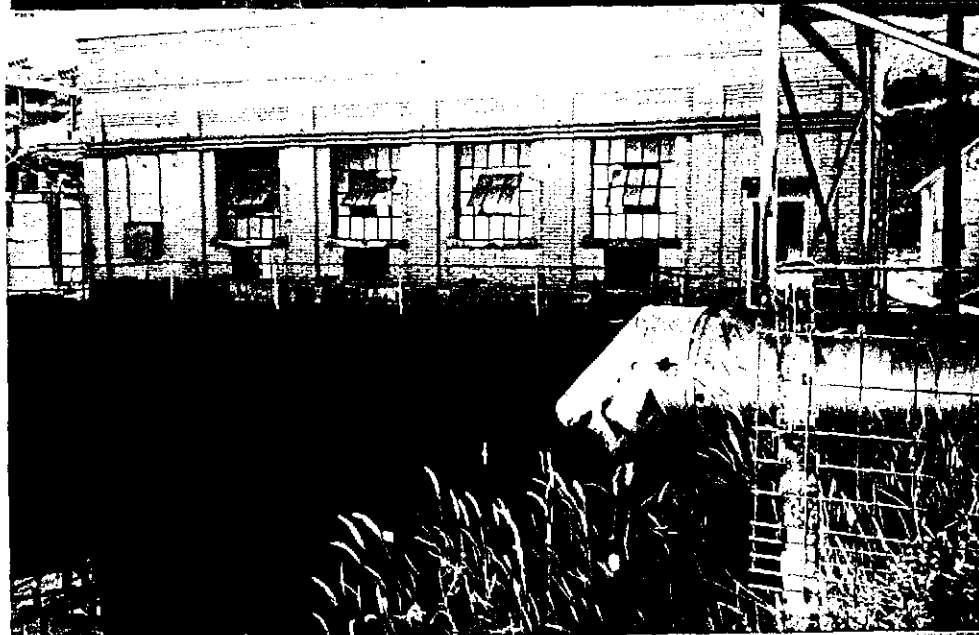
← waste water overflow
