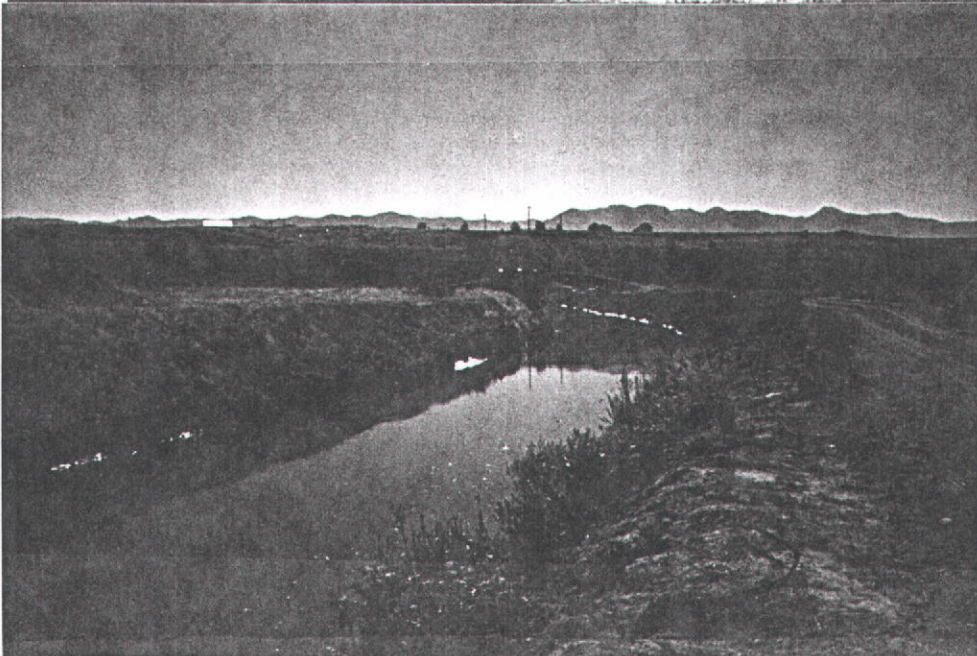
Canal from Bear River to pump station
