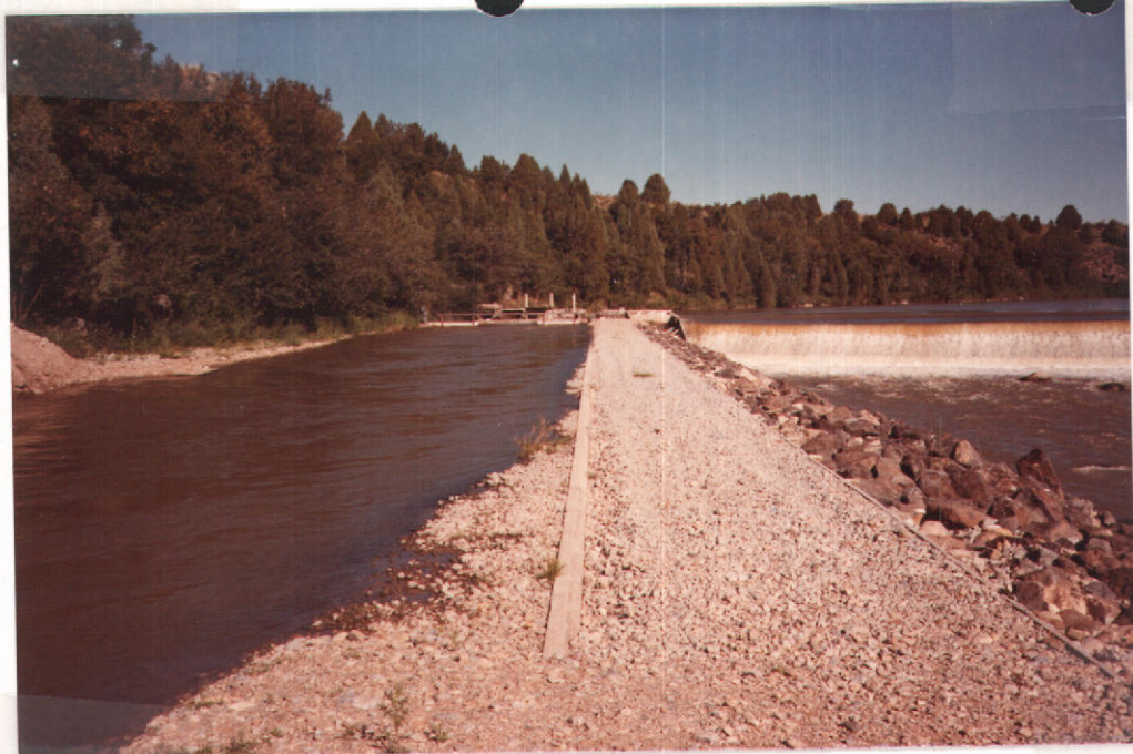
LAST CHANCE DAM AND CANAL
