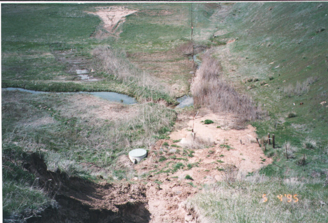
VIEW OF NORTH WELL
