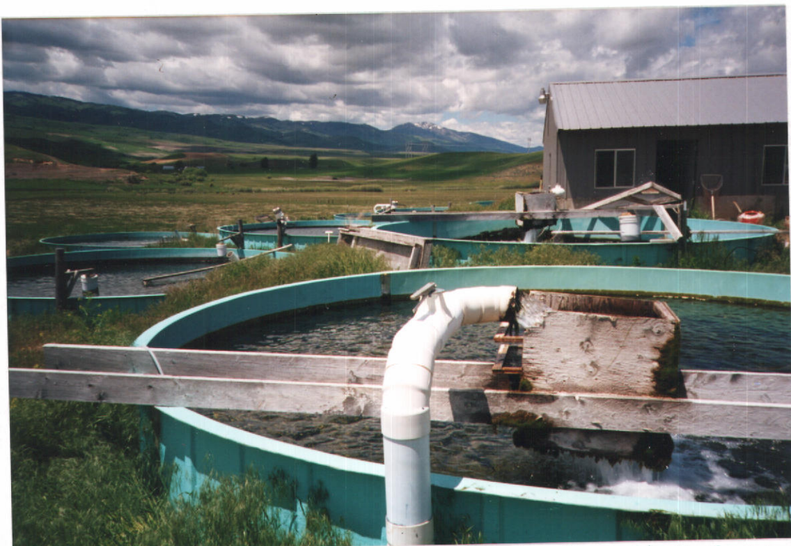
Inlet to first of holding tanks looking North By West
