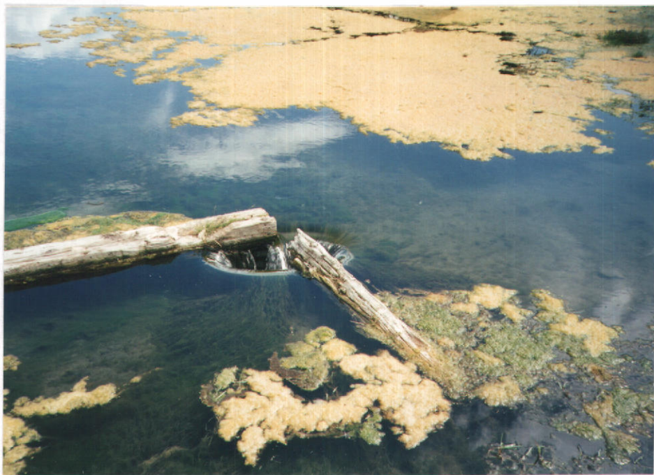
Photo showing the outlet of the pond.
