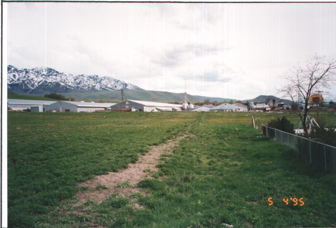
VIEW OF PLANT FACILITIES PLACE OF USE
