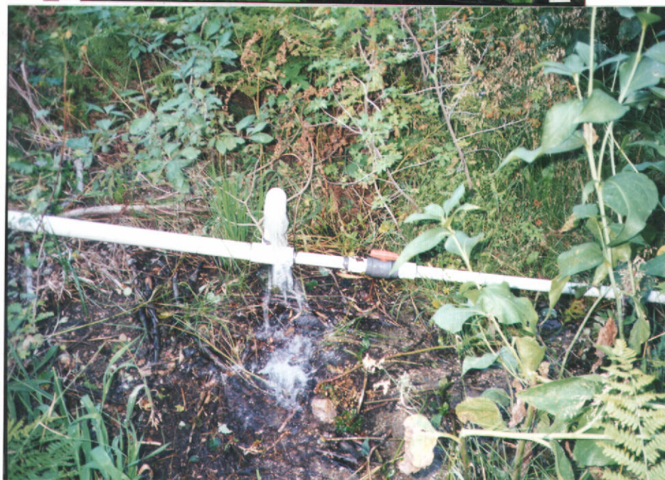
End of 4" PVC Pipe with overflow Spring is to the left approx 500 ft looking North. Cabin to the right at 50 ft.
