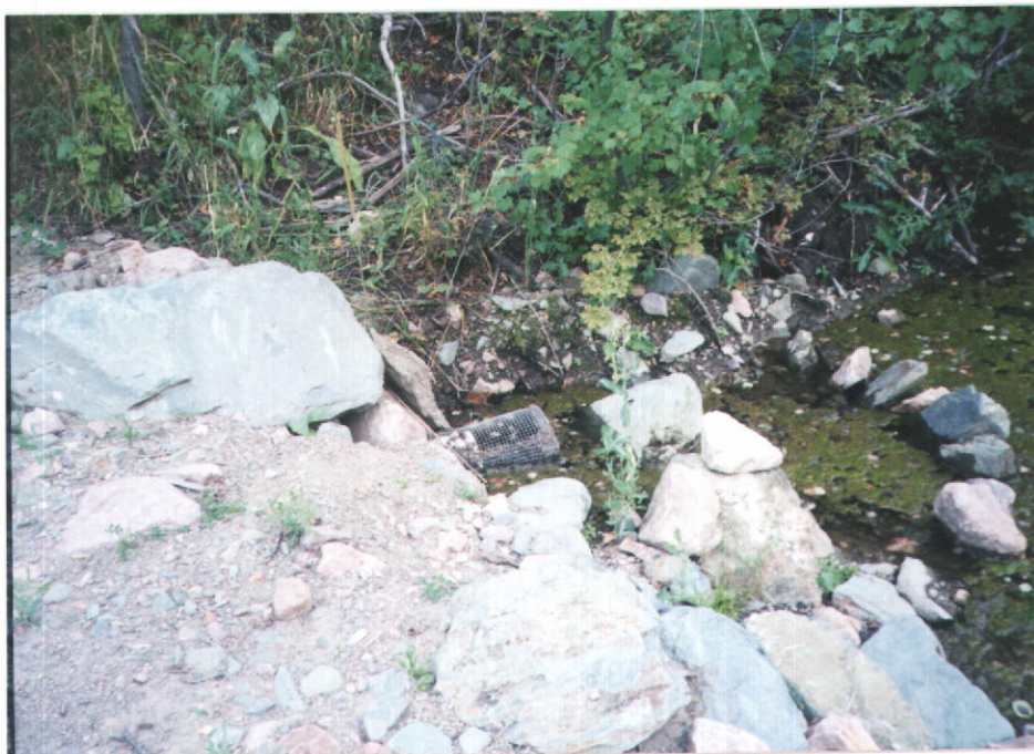
outlet of pond - looking South
