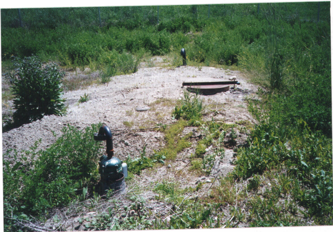
13-07529 Well #2 Looking North West
