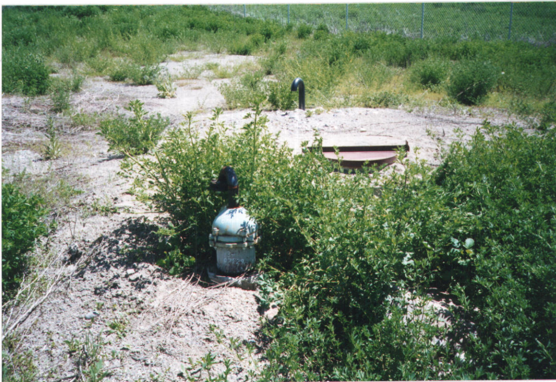
13-07529 Well #3 with underground bunker Looking South.
