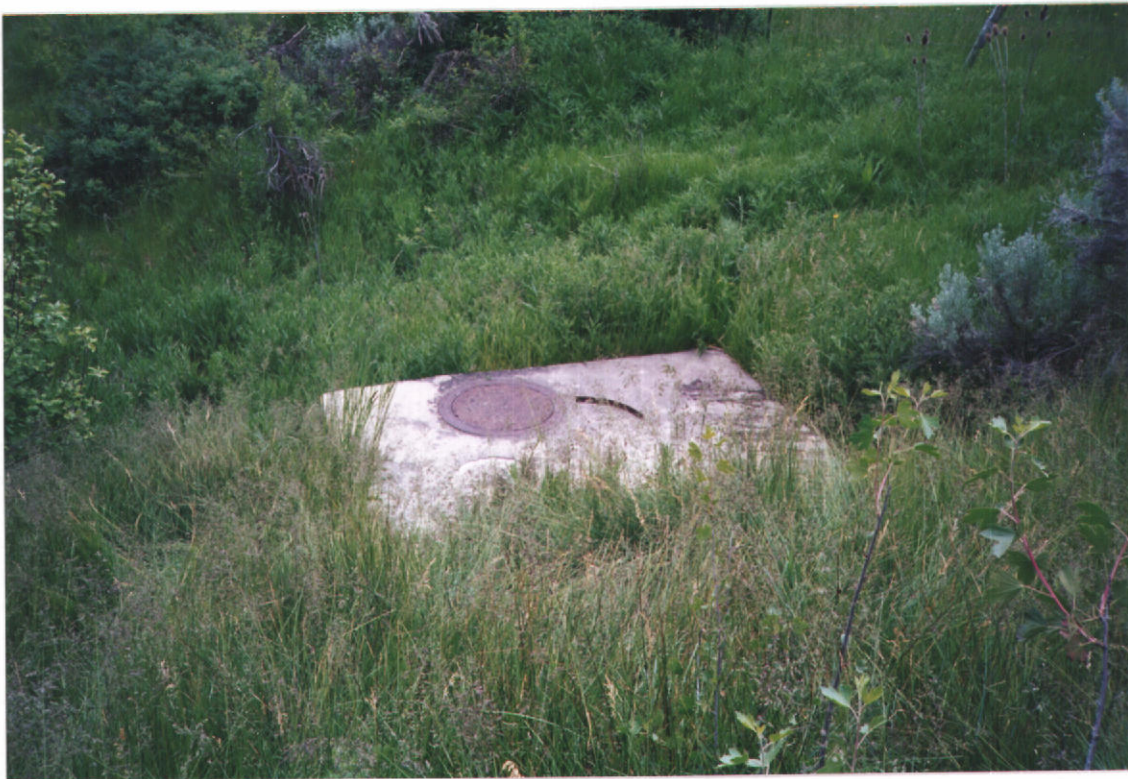
13-07544 Concrete Collection box. Springs are piped in from Right and South in Top Looking South
