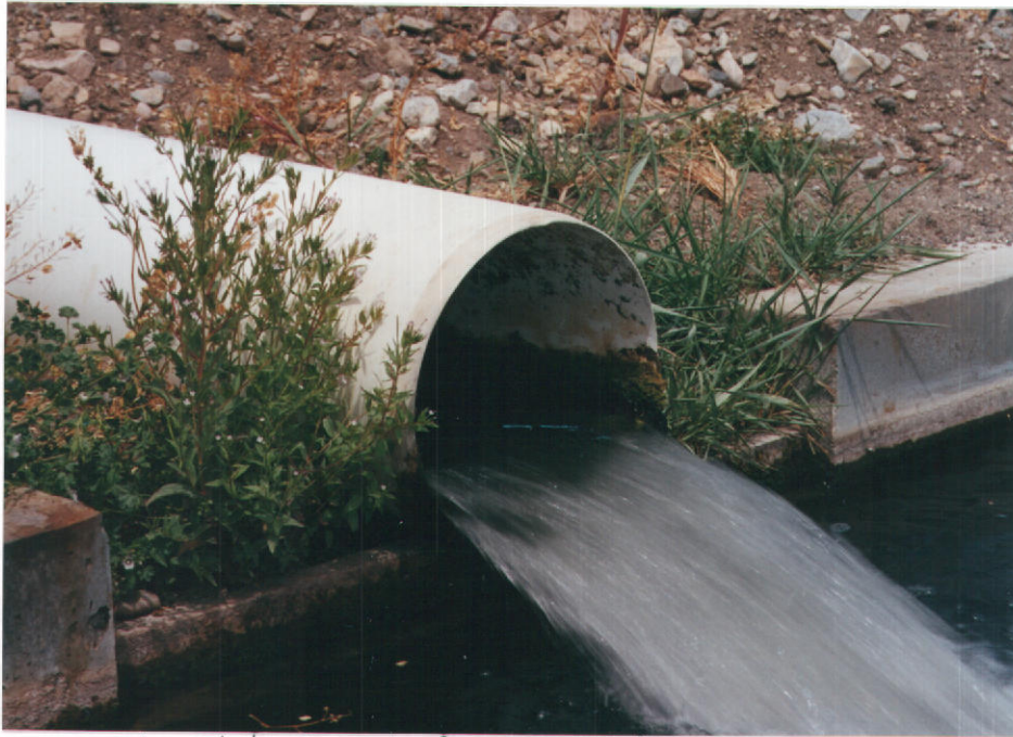
# 13-7561 Photo doesn't show it well, but water line in pipe is a good inch lower than it has been earlier in the year. Flow shown coming into tank #4
