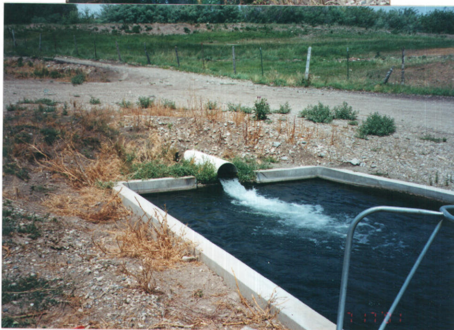
13-7561 Water entering tank 4
