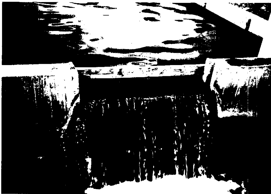
# 13-7561 Weir between tanks
