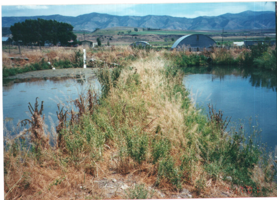
# 13-7561 Two settling ponds
