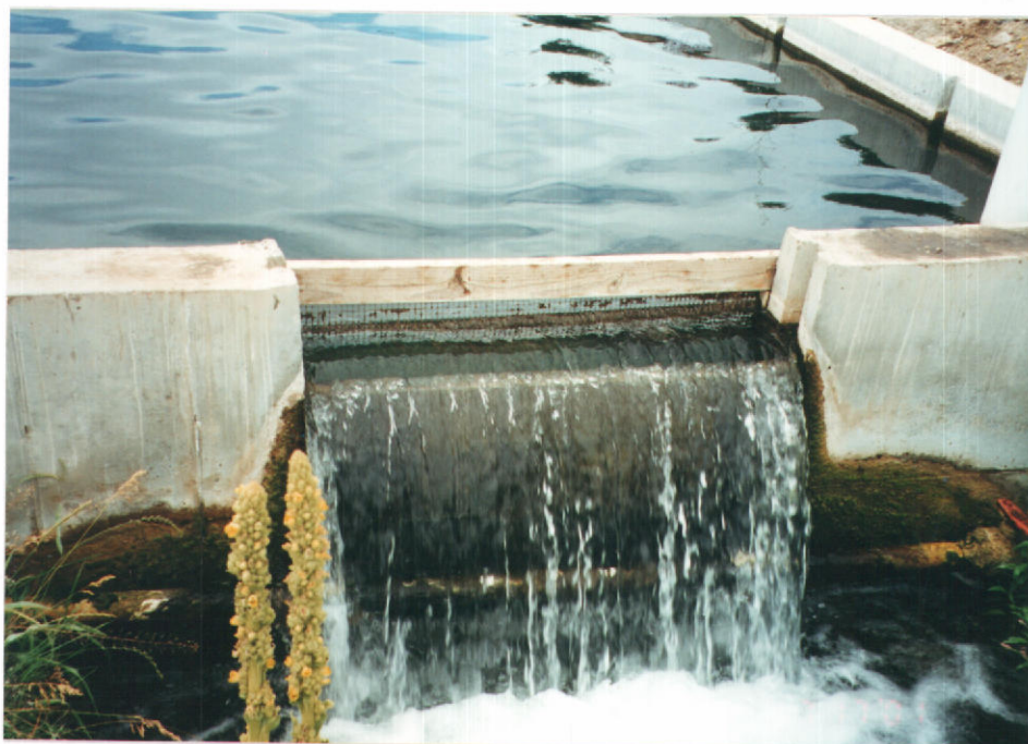
# 13-7561 Weir between tanks
