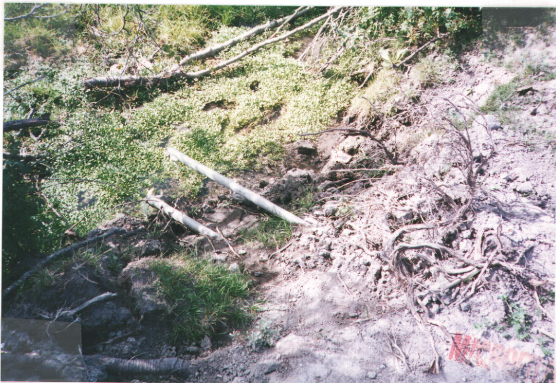
Blow off lines
