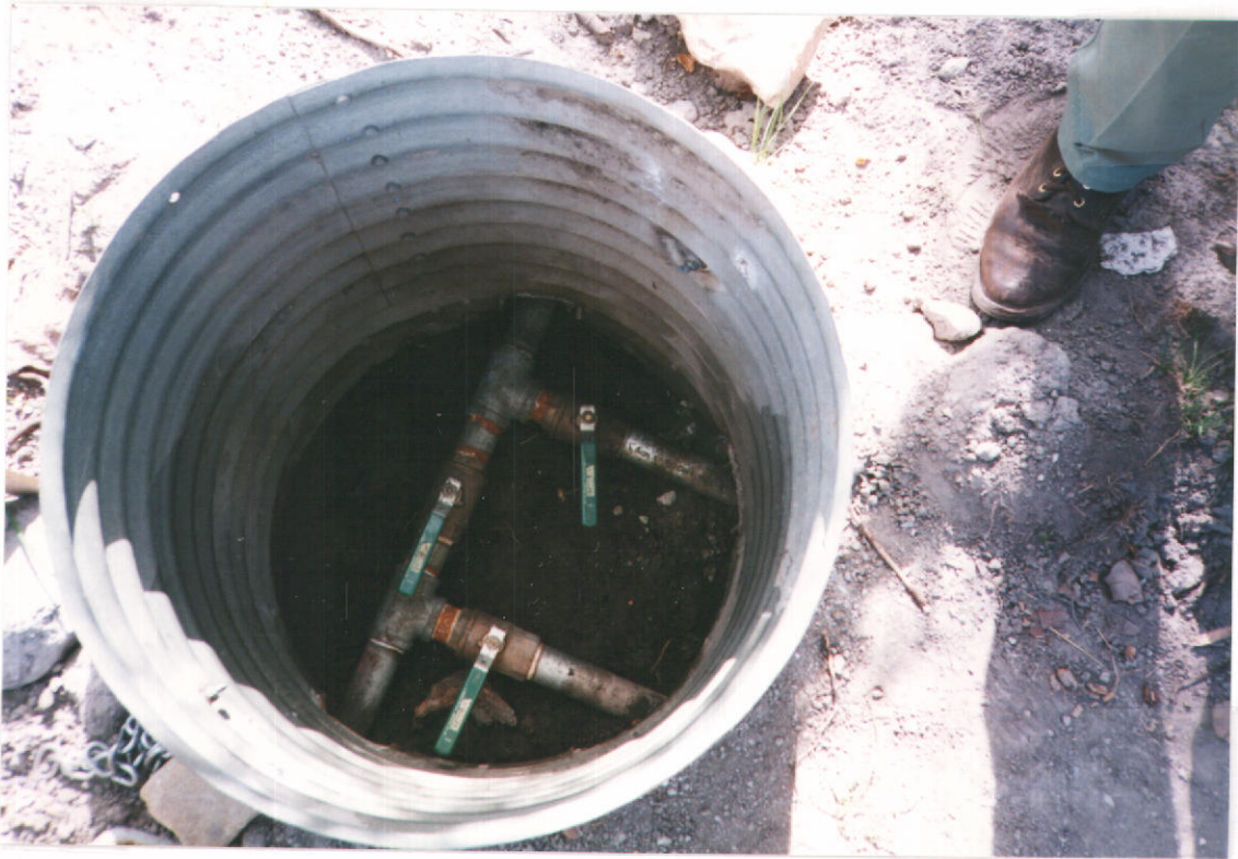
Vertical Culvert housing
