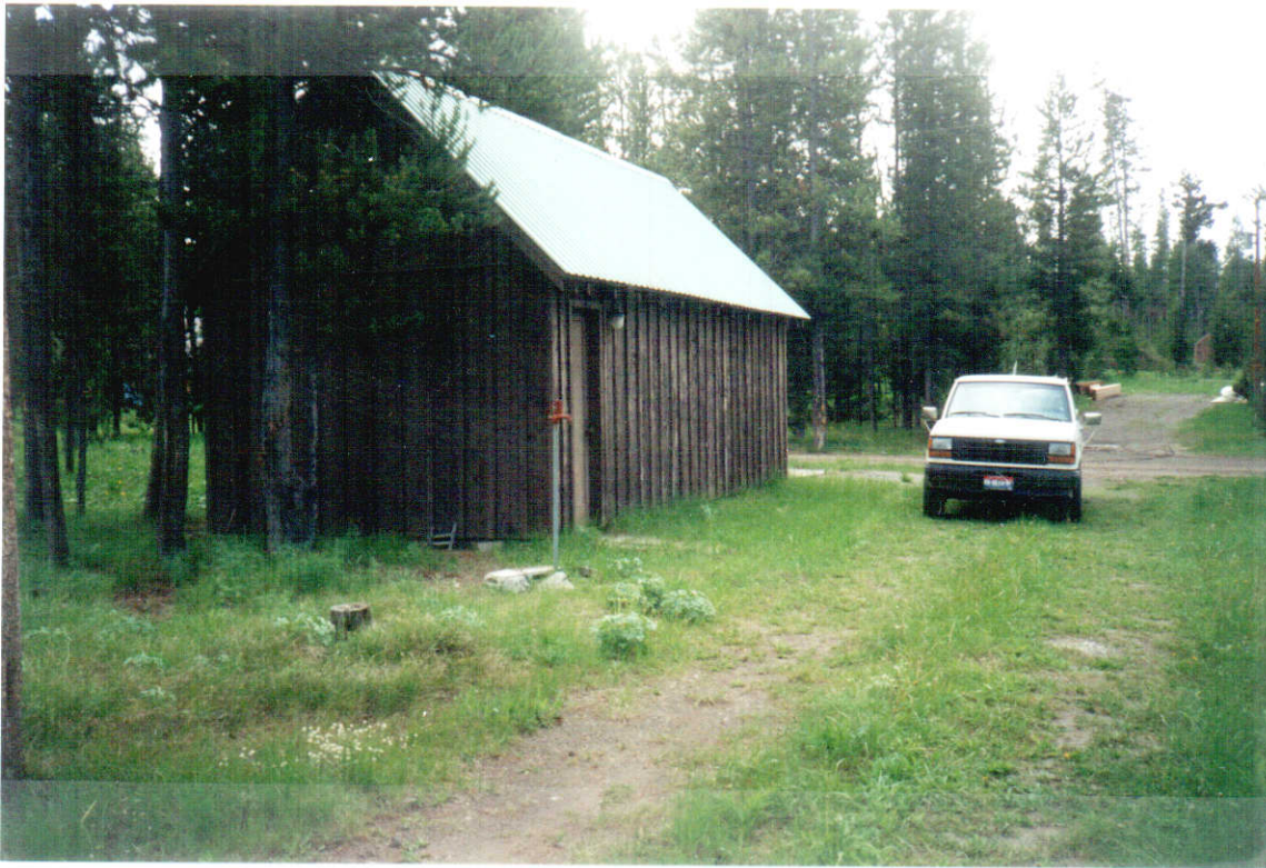
Fig. 1 - Point of diversion inside garage.
