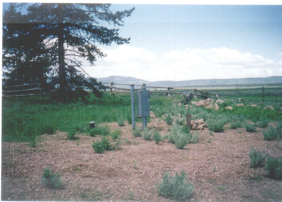
Fig. 1 - Point of diversion and control box.
