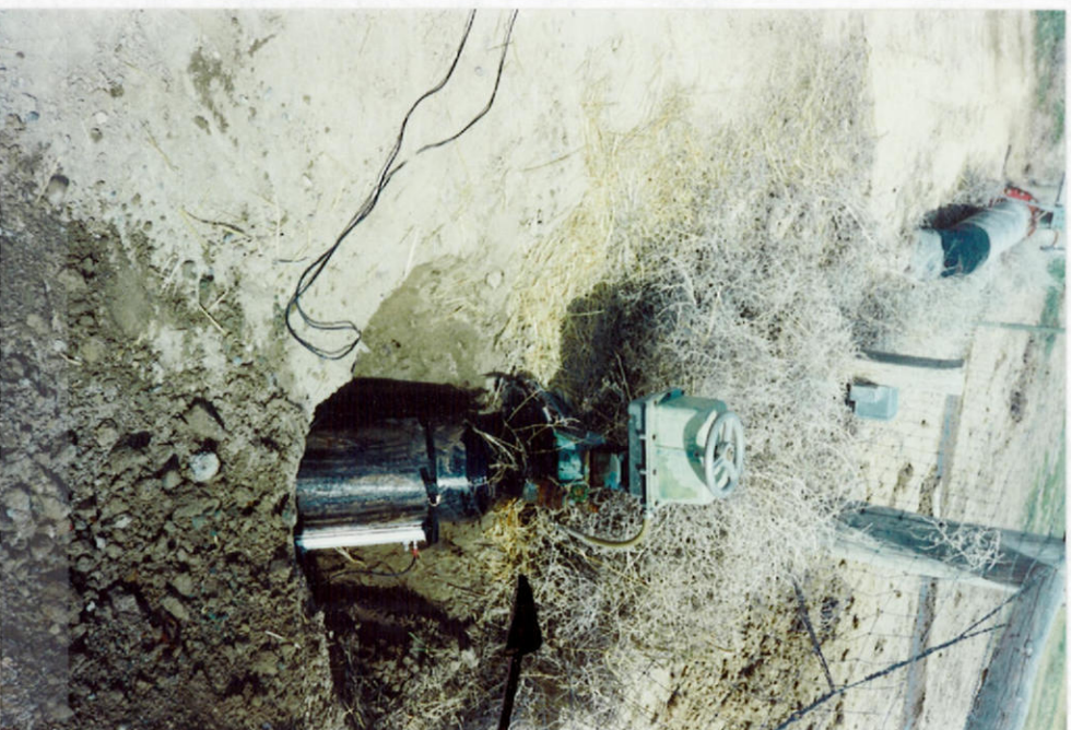
SOUTH - RUNNING MAINLINE
