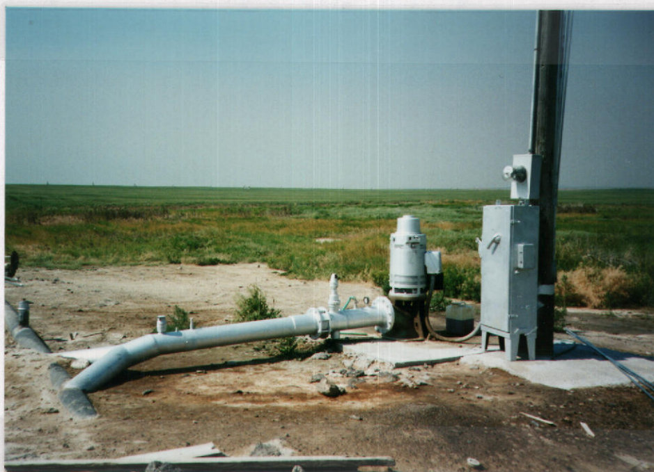
Fig. 2 - Point of diversion looking southwest.
