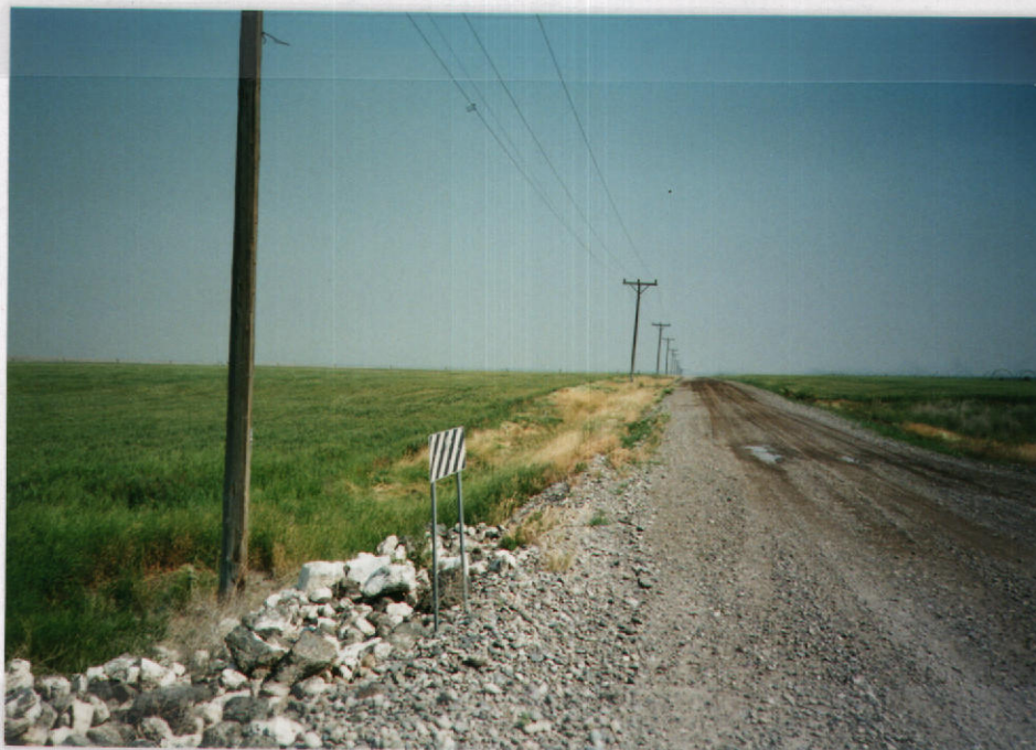
Fig. 4 - Place of use from point of diversion looking northwest.
