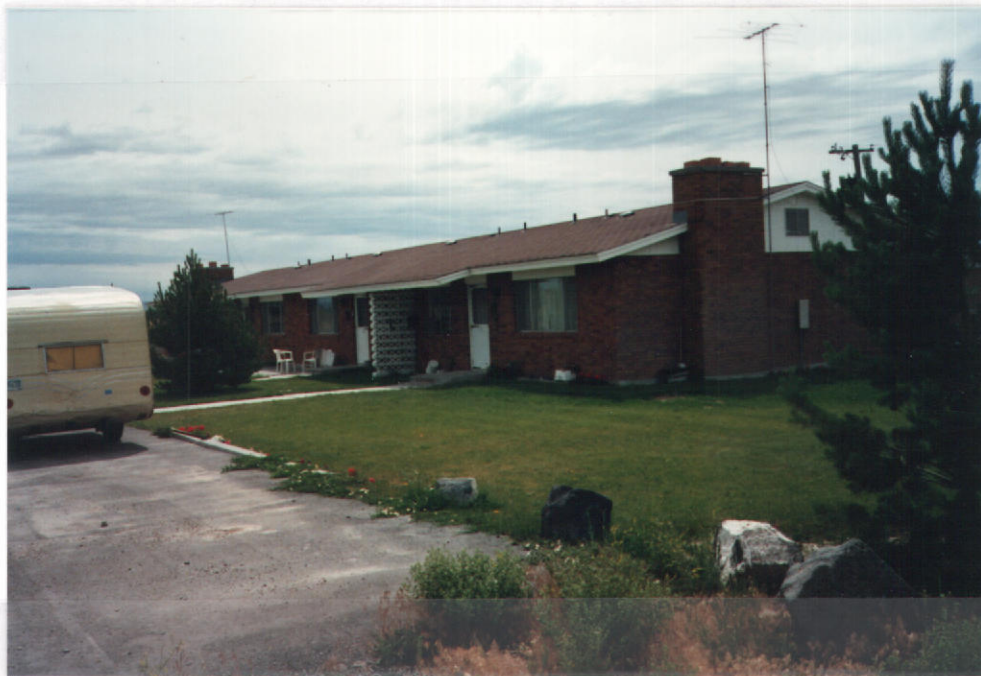
Fig. 3 - Four-plex apartment looking southeast.
