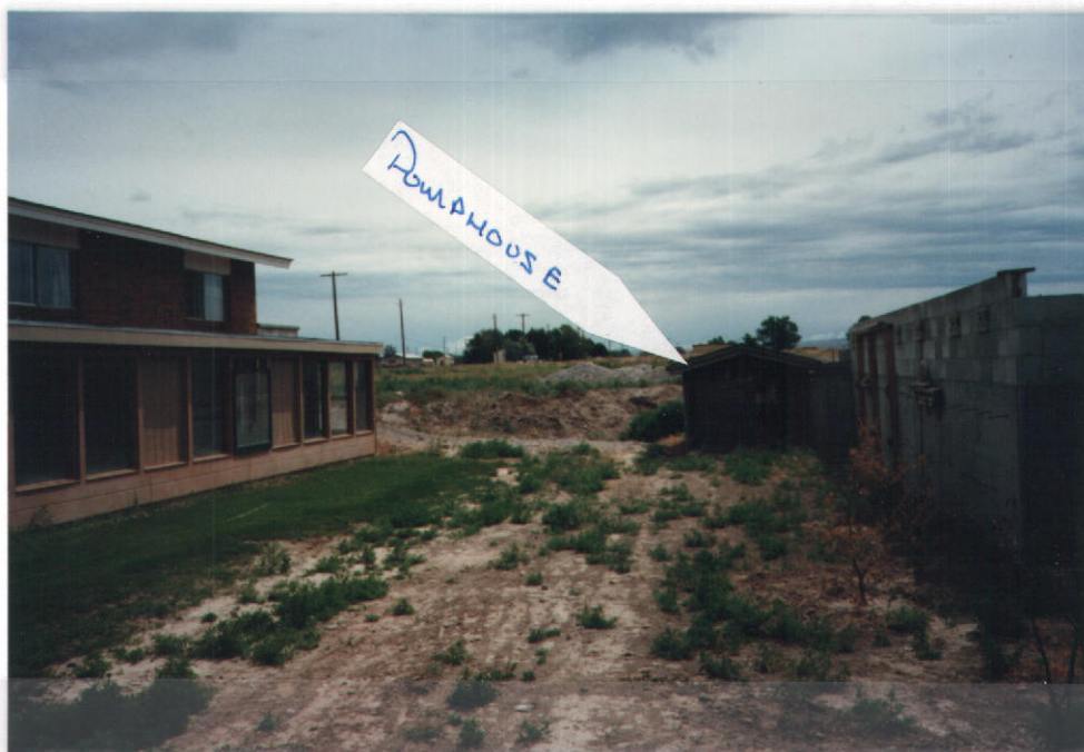
Fig. 4 - Garden area behind apartment showing pumphouse.
