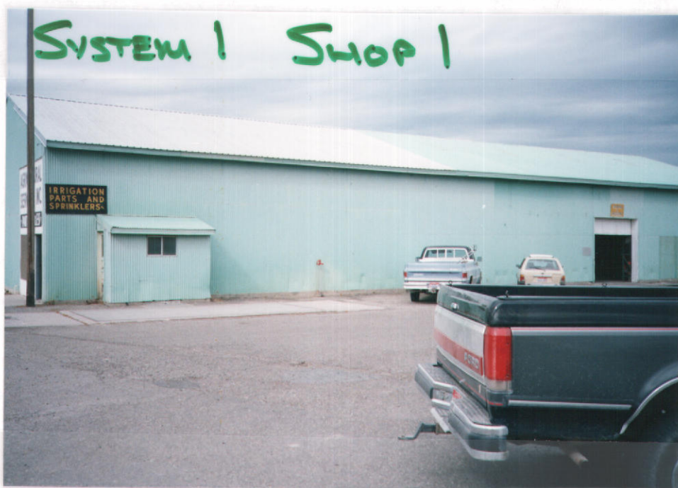
Fig. 3 - Shop building #1 served by "System #1".
