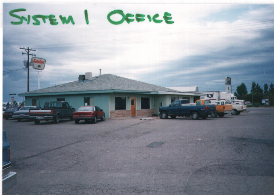
Fig. 2 - Office building served by "System #1".
