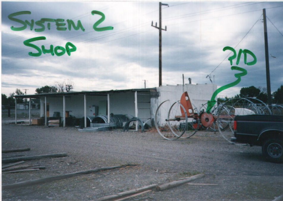
Fig. 5 - Shop building served by "System #2".
