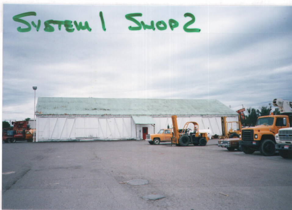
Fig. 4 - Shop building #2 served by "System #1".
