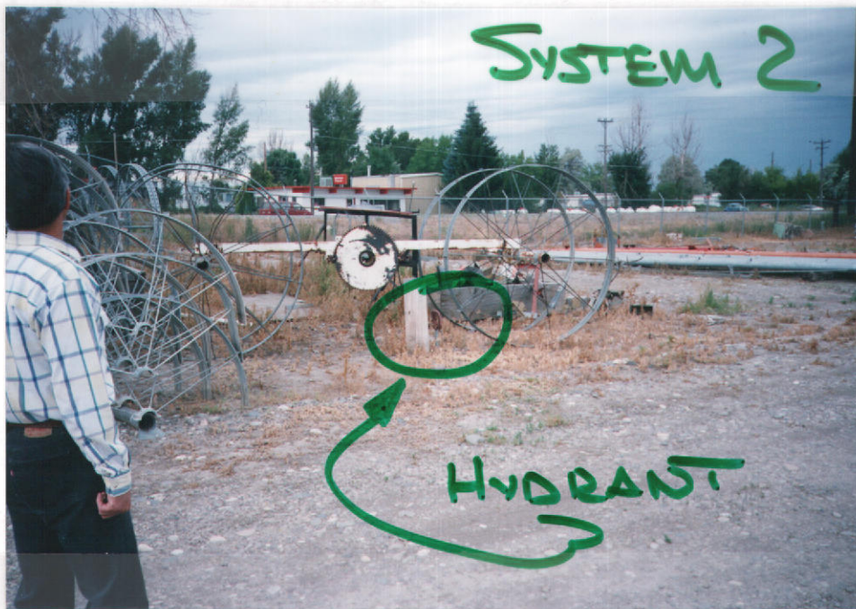
Fig. 6 - Hydrant served by "System #2".
