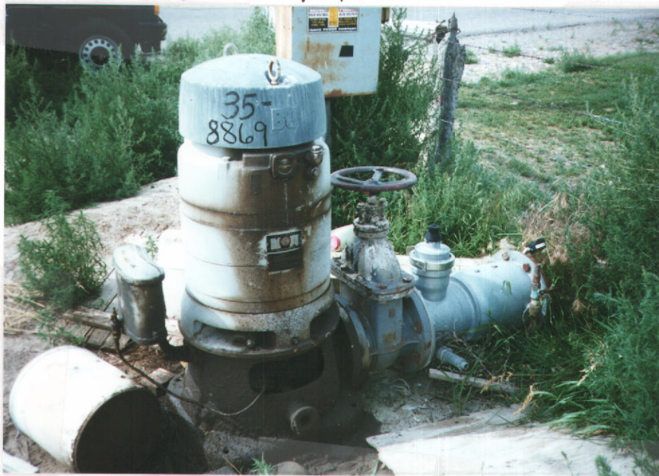
Point of Diversion
