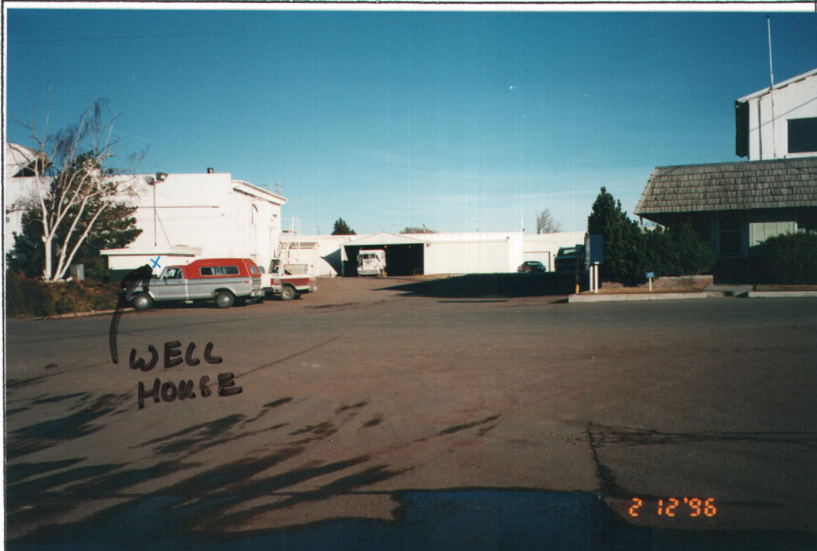
VIEW OF PLANT (PARTIAL)
