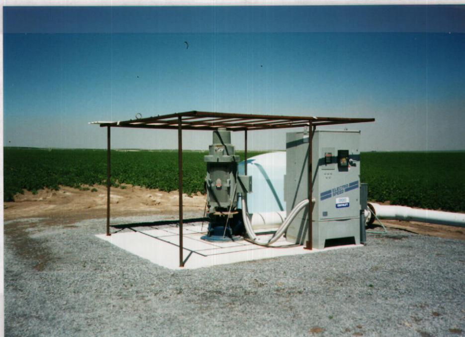
Fig. 2 - Complete diversion system.
