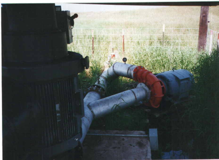
Plate 2 - Booster assembly from motor and pump.
