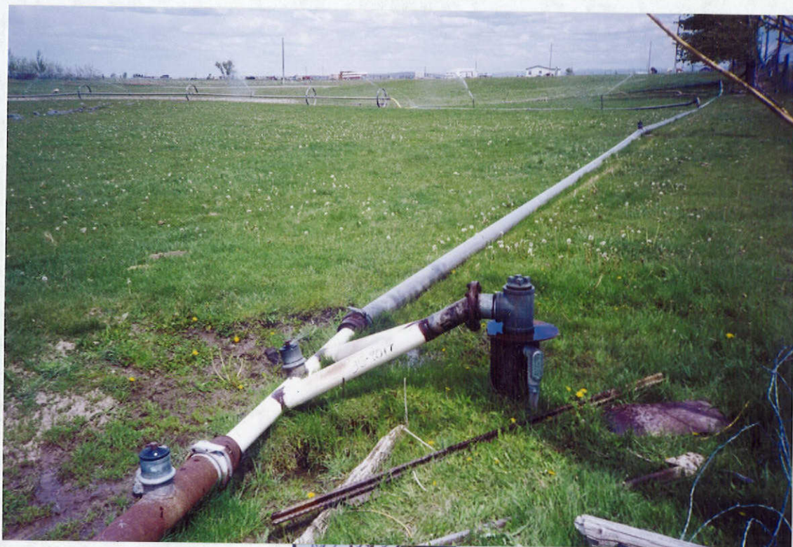
POINT OF DIVERSION VIEW E-NE
