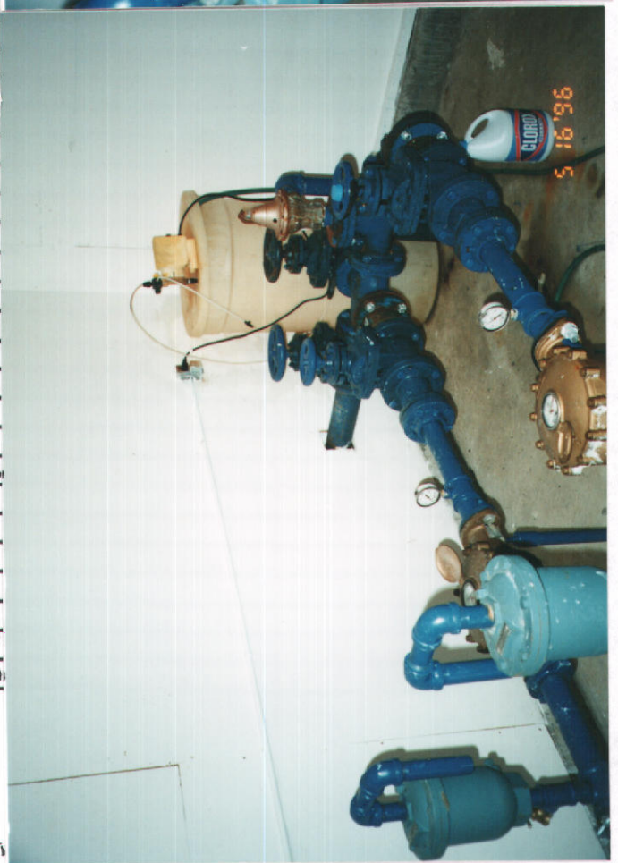
Well Head Valves & Flowmeters
