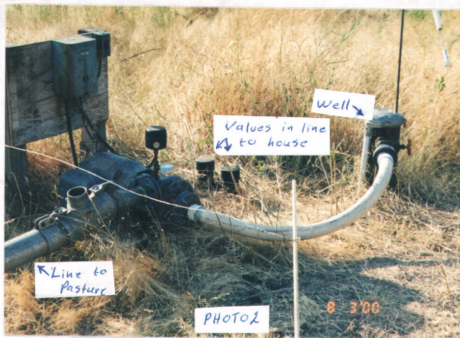
Photo 2. Showing well, booster pump, and diversion.
