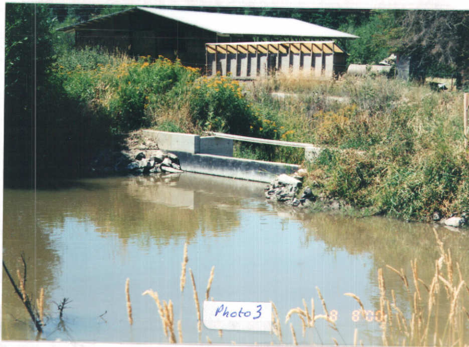
Photo 3. Dam and spillway.
